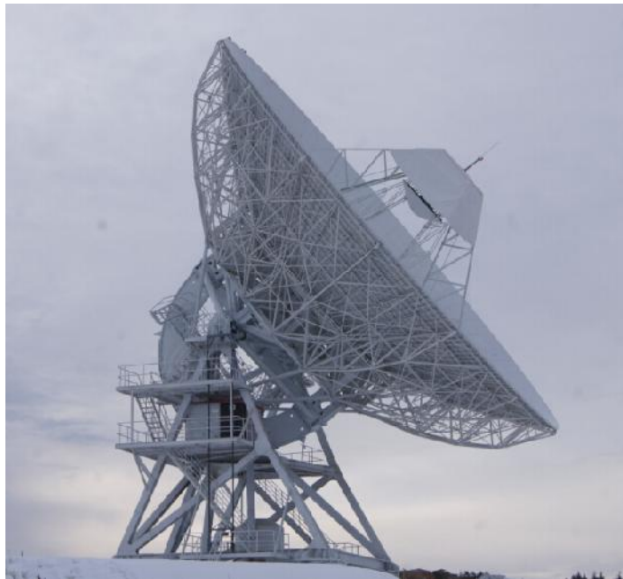
Figure 1. Newly painted 26m antenna at Nanshan
