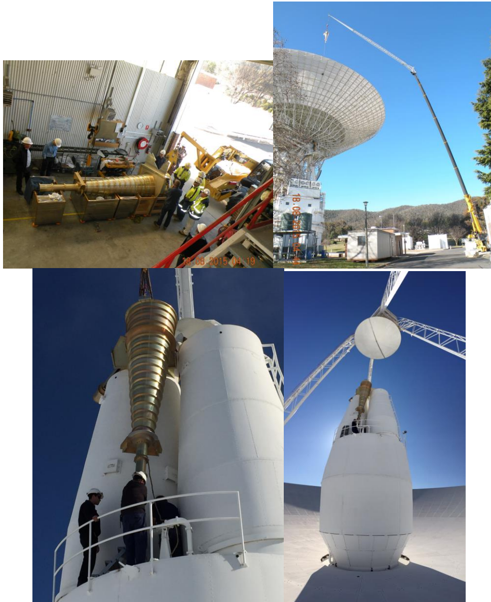
Figure . Details of the installation of the new L-band feed in Canberra, 70m antenna DSS-43.
